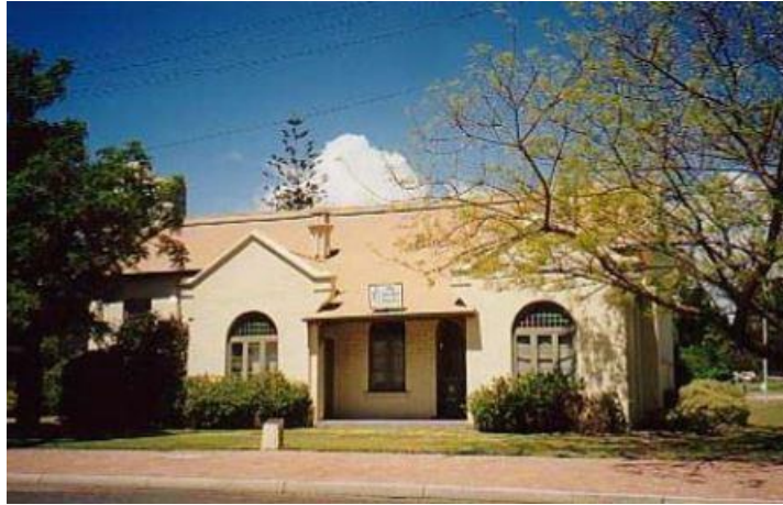
Mechanics Institute Hall completed in 1899 (now known as the Old Mill Theatre ) South Perth (South Perth Municipal Heritage Inventory place MPt5)
